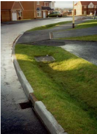
Road side swale
