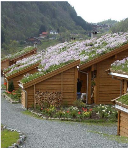
Green roof in stormwater management
