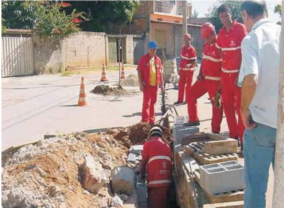
Figure 5 Installing a gully with permeable bottom, at Vila Guaratã
