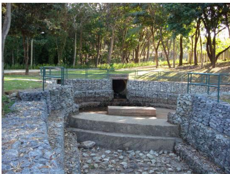
Figure 9 Existing gabion and concrete structures in the Lagoa do Nado Park
