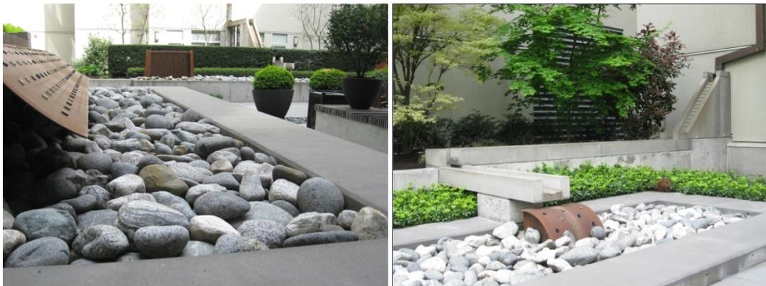
**Fig. 4. A system of concrete cascades, river stone filled basins and Cor-Ten steel weirs manages all rainwater at 10<sup>th</sup>@Hoyt Street Apartments in Portland on site (© J. Hoyer).**
